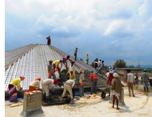
Mesh placement and RCC work
