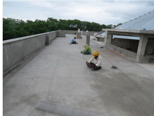
Terrace shielding with SS mesh
