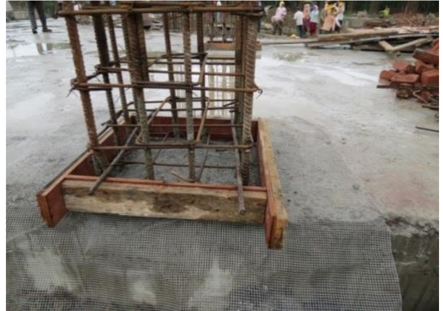
SS mesh brought down at plinth level
