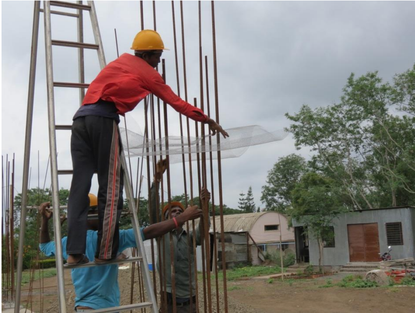
SS mesh inserted in the pillar
