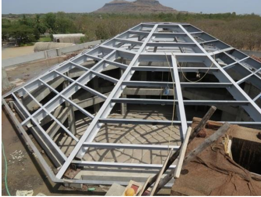
Installation of Dome structure
