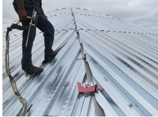
Placement of GI sheets
