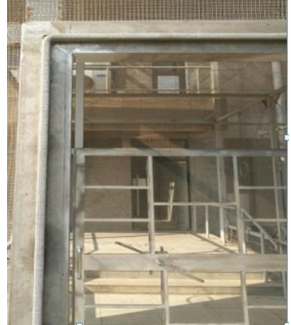
Shielded Gasket on door frames with U groove on door
