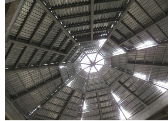
Bottom view during installation
