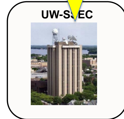
Data Processing Center
