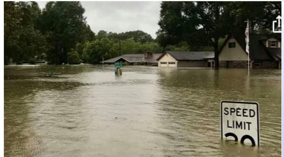
Flooded roadway in Marshall. (Marshall, MO Fire Department)
