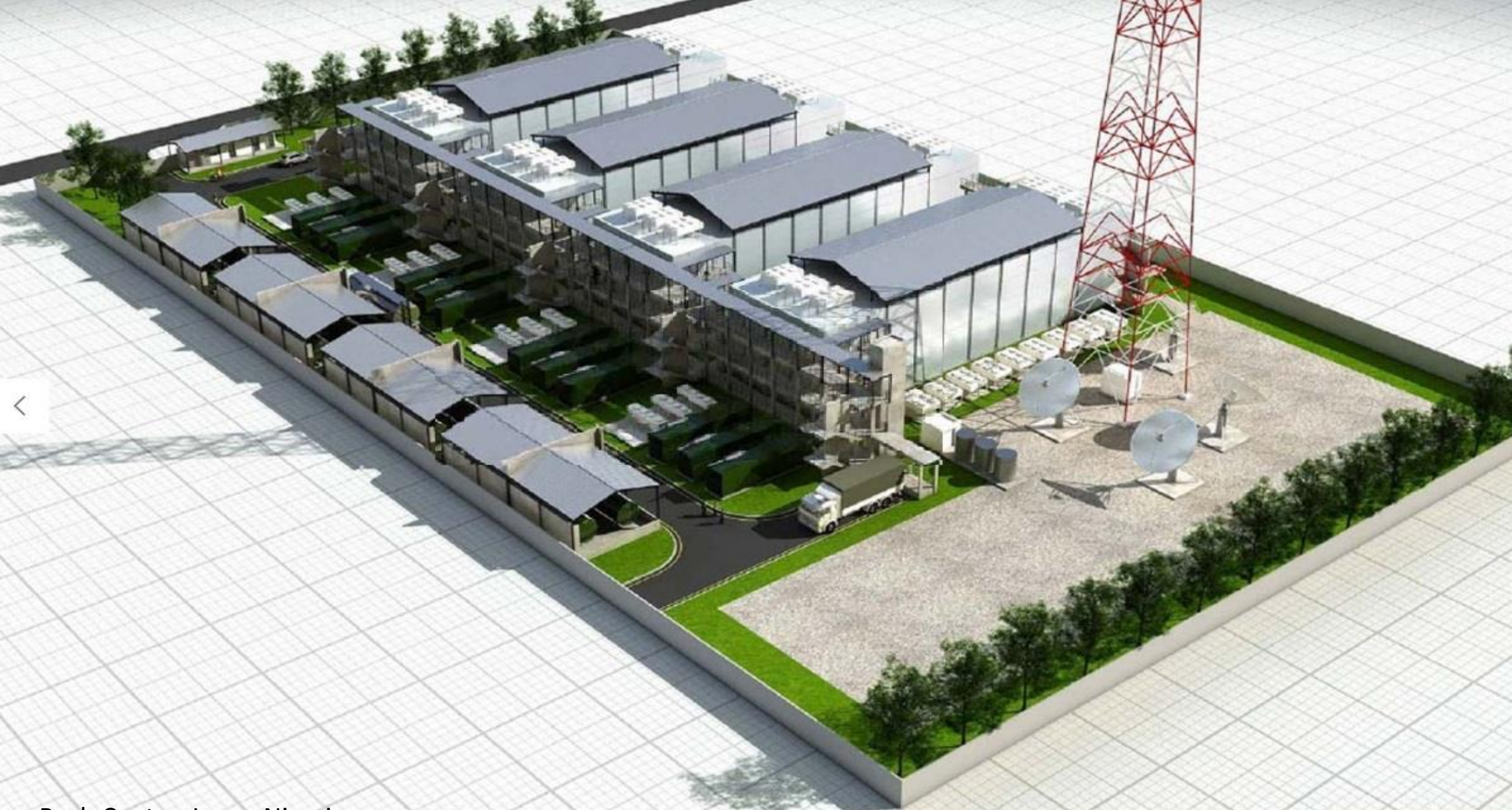
Rack-Centre, Lagos Nigeria
